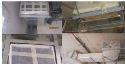
Upon installation, seal all permanent ducts and vents to minimize contamination during construction. Remove any seals only after all phases of construction are completed.
